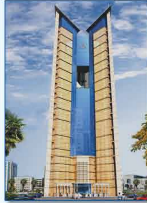
Sharjah Islamic Tower Headquarter
